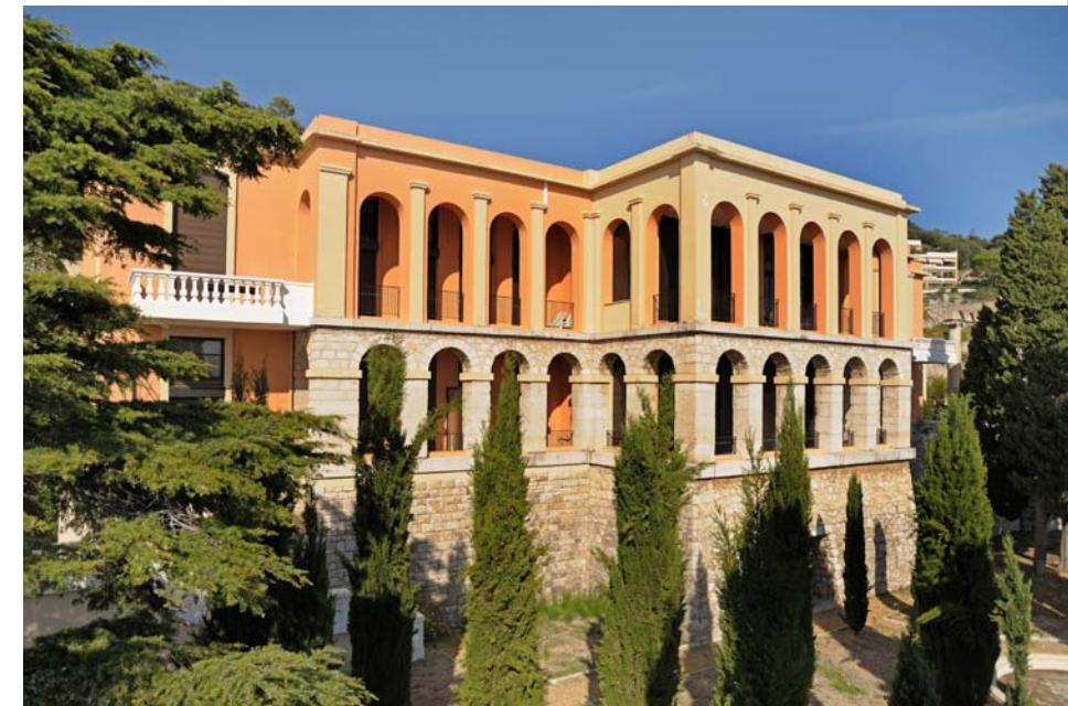
Burger Sotheby's International Realty recorded the € 48 million sale of the legendary Palais Maeterlinck
