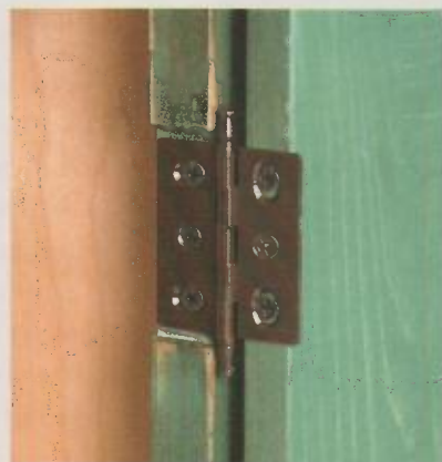
Traditional butt hinge. A furniturelike hinge on this door is set into a mortise in the frame.
