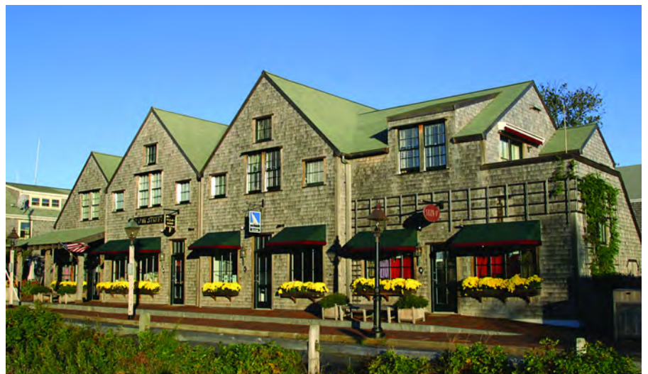
The recently expanded Windwalker Offices at 12 Oak Street.
